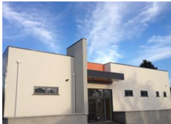
Tullow and South Leinster Tennis Club, Co. Carlow.
